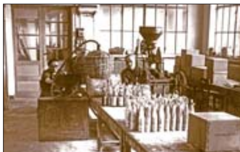
31. Balance (France). Plant for production of biphosphate.
