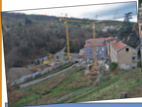
60. Renovation work. Notre Dame de l’Hermitage (2008).
